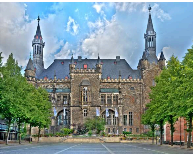
Aachen City Hall/The coronation hall is on the first floor of the building. Inside you can find frescoes which show legendary scenes from the life of Charles the Great as well as Charlemagne's signature.
